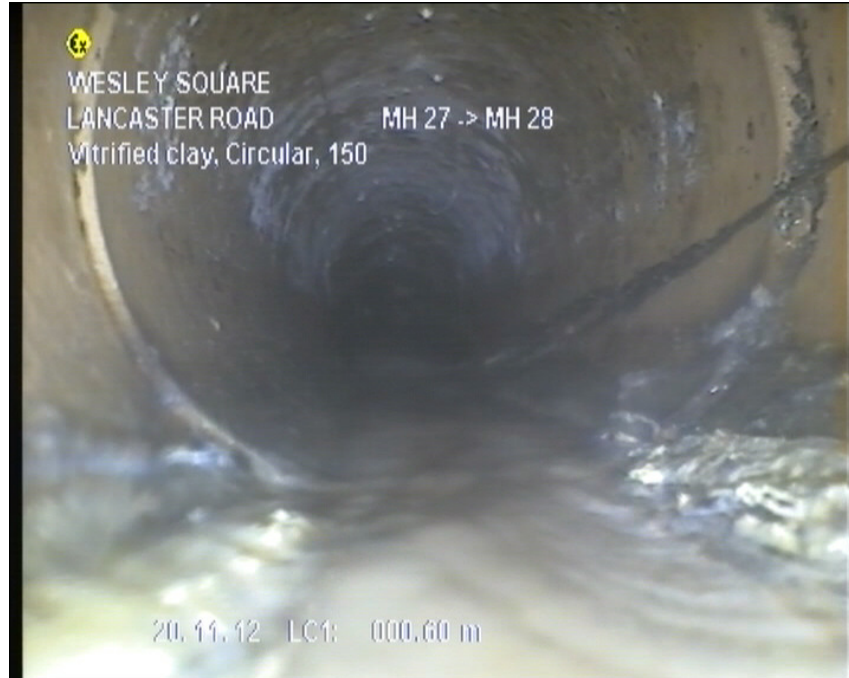
Photo: 55_4A 0.6m, Fine Roots at joint
