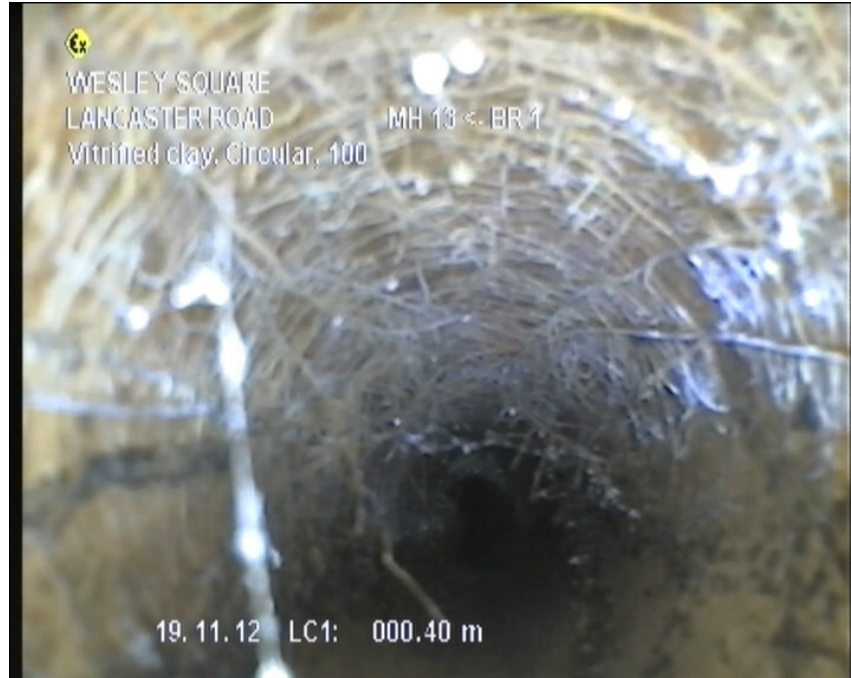
Photo: 32_4A 0.4m, Mass Roots 10 % cross-sectional area loss
