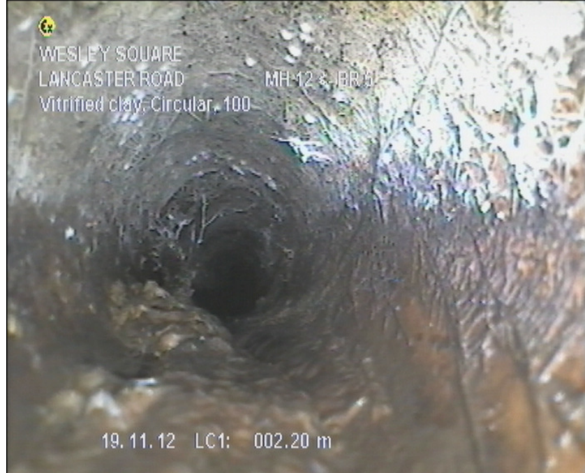
Photo: 159_4a 2.2m, Mass Roots 10 % cross-sectional area loss
