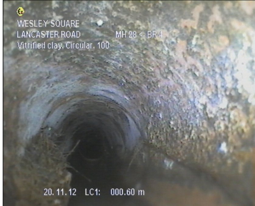
Photo: 582_4a 0.6m, Mass Roots 20 % cross-sectional area loss
