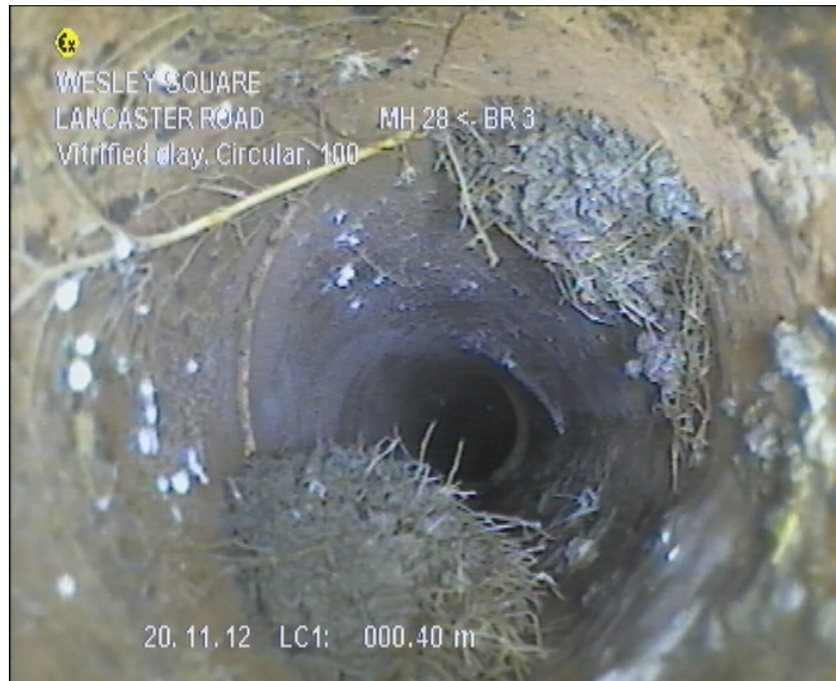
Photo: 571_5a 0.4m, Mass Roots 20 % cross-sectional area loss
